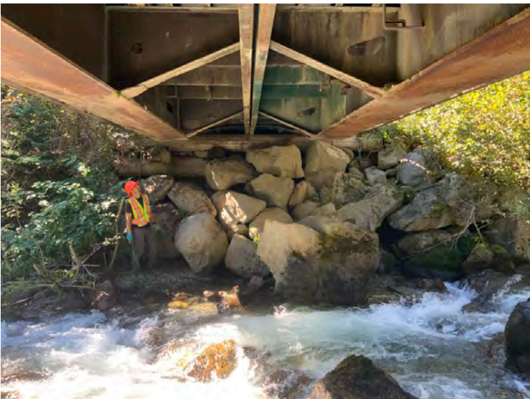
Right Bank Abutment when facing downstream
