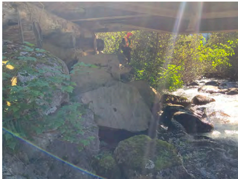
Left Bank Abutment when facing downstream
